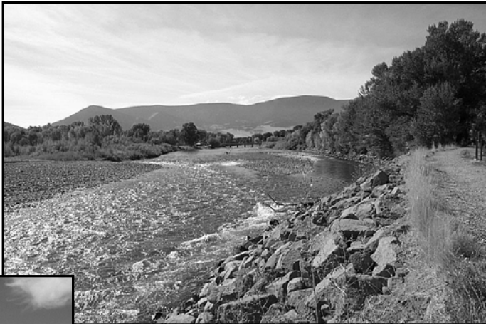
Photo 65. Livingston levee with low water. Photo by E. Galli-Noble.
